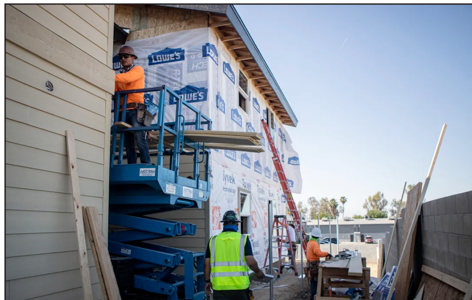
Workers build affordable housing in Bakersfield on May 29, 2024. Californians will vote on an affordable housing bond issue in November.
